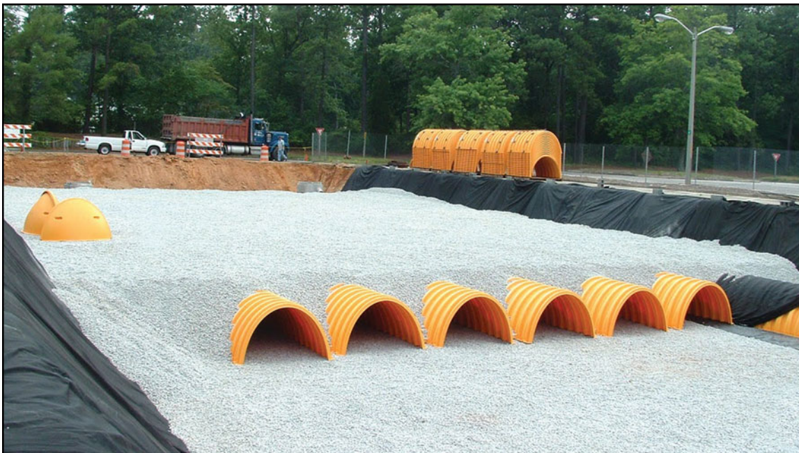
Image 3: Installation of underground stormwater Stormtech™ arched chamber system
